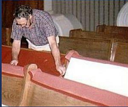
Step 3 Pull fabric over backs & attach
